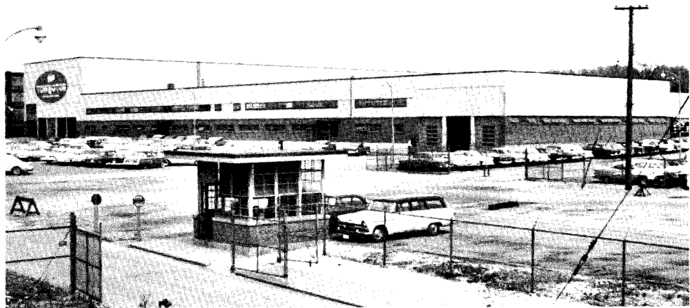
The Noble Road Plant was constructed in the mid '50s adding 155,000 square feet of space.
