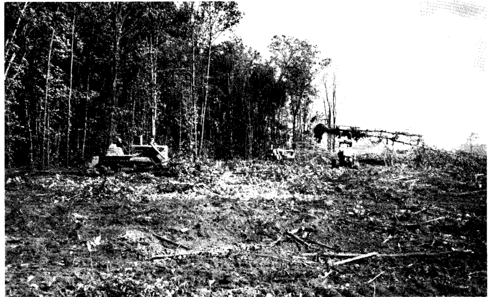
Ground clearing operations began in 1966 for the construction of the Mentor Plant.
